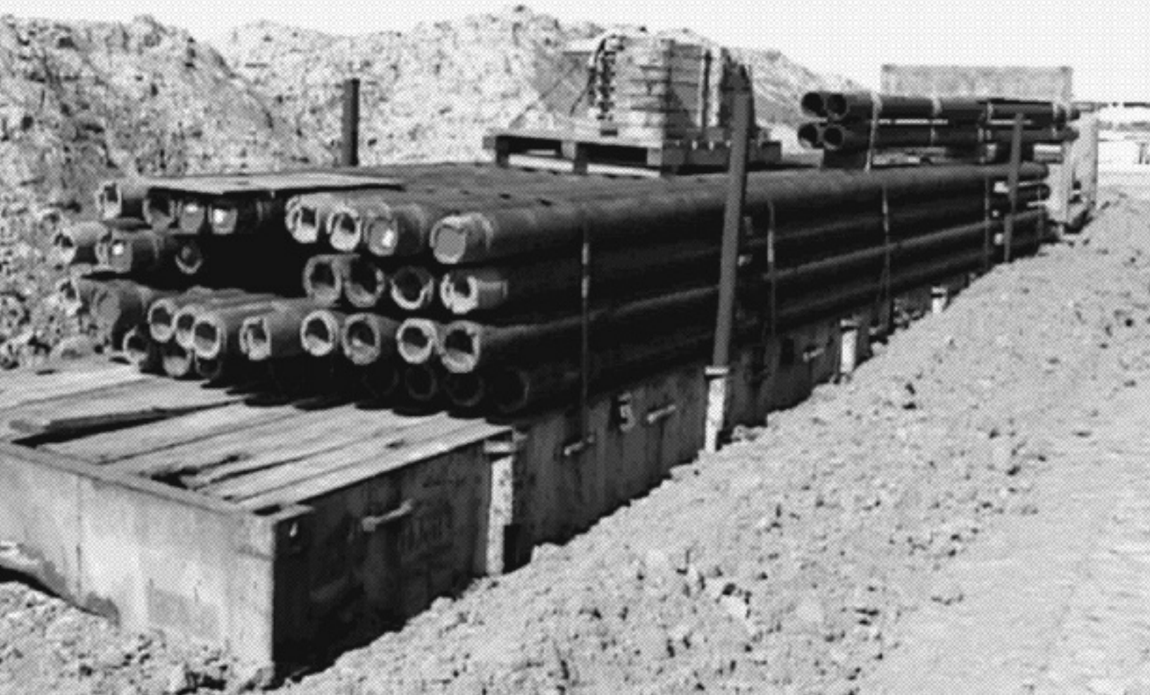
Pipes await Halliburton crews at Al Fathah crossing, Northern Iraq, Photo: U.S. Army Corps of Engineers video
